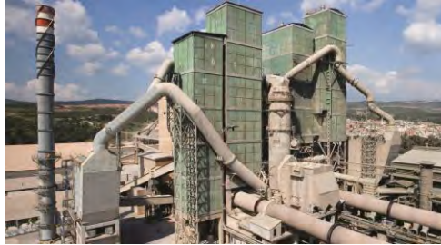
Construction of Vertical Raw Mill at İzmir Batıçim Cement Factory
