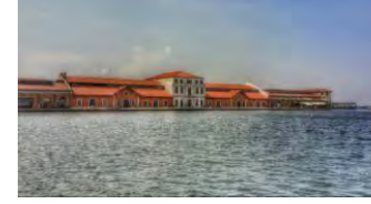
Construction of Konak Pier Shopping Mall
