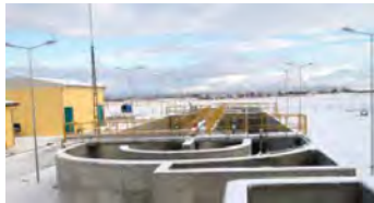
Afyon Çay Municipality Wastewater Treatment Plant
