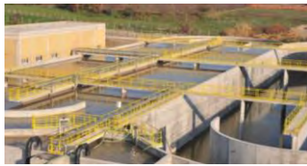
Kemalpaşa Organized Industrial Zone Industrial Wastewater Treatment Plant
