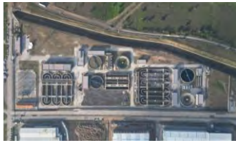
Design and Construction Works of the Manisa Organized Industrial Zone Phase III Wastewater Treatment Plant
