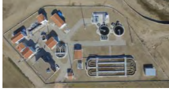
İzmir Metropolitan Municipality İZSU Bayındır Hasköy Wastewater Treatment Plant
