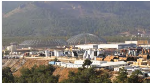
Construction of Mersin Medcem Cement Factory
