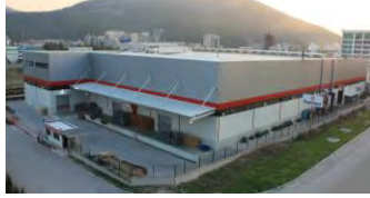
Süperpar Factory Construction
