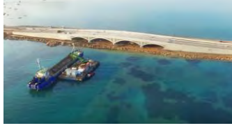
Construction of the Ayvalık Lale Island Access Bridge
