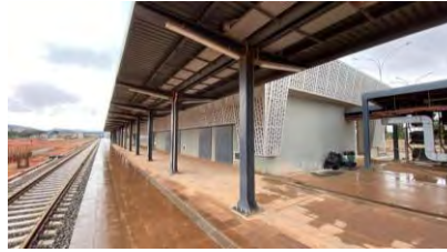
Construction of Railway Line Structures between Morogoro and Makutupora in the United Republic of Tanzania
