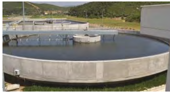
İzmir Metropolitan Municipality İZSU Doğanbey Wastewater Treatment Plant
