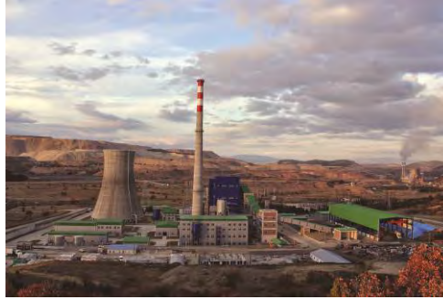
Construction of Kütahya Tunçbilek Thermal Power Plant
