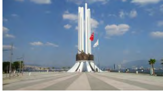
Construction of the Women's Rights Monument in Karşıyaka, İzmir
