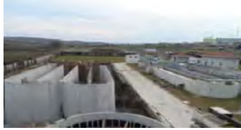
Balıkesir Organized Industrial Zone Chemical Wastewater Treatment Plant
