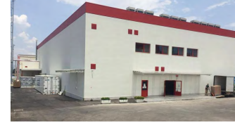
Construction of the Vestel Kitchen Appliance Factory
