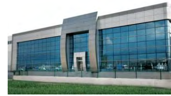
Construction of the Motorcu Hayri Factory
