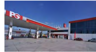
İleten Deri Fuel Storage and Distribution Facility
