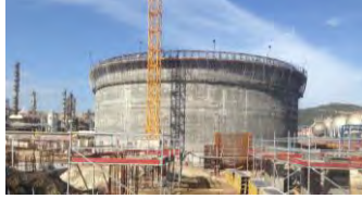
Construction of the SOCAR Equalization Tank
