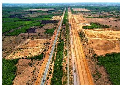
LOT 3 MIT Earthworks and Civil Structures Project in the United Republic of Tanzania
