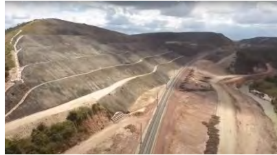
Earthworks for the Railway Line Construction between Dar es Salaam and Morogoro in the United Republic of Tanzania
