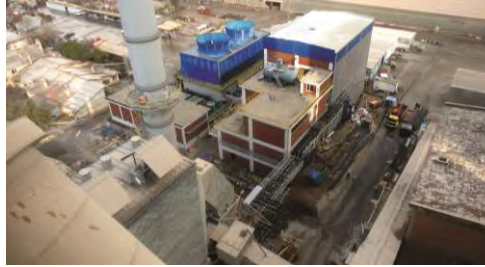
Construction of 12 MW Waste Heat Recovery Power Plant at İzmir Batıçim Cement Factory
